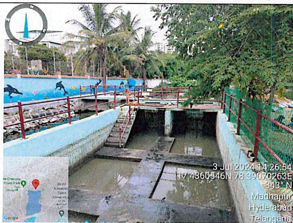
Durgam Cheruvu interception and diversion structure
