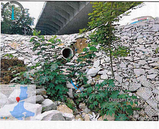
Durgam Cheruvu storm water drain inlets
