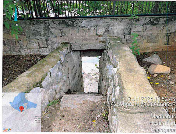
Durgam Cheruvu sluice area
