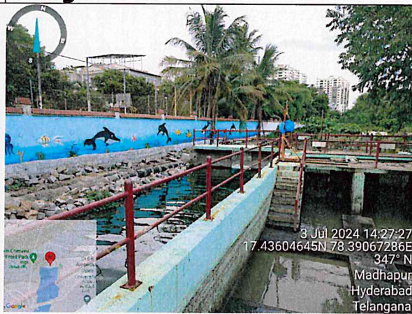
Durgam Cheruvu interception and diversion structure
