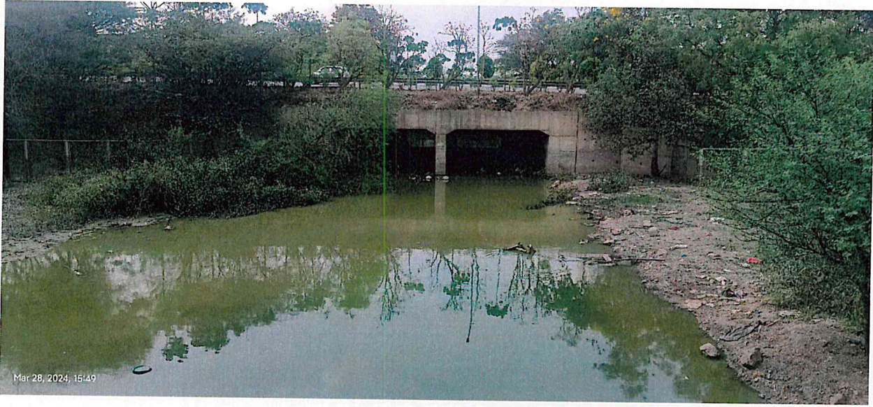
Inlet drain joining into Chinnadamara cheruvu near ORR service Road
