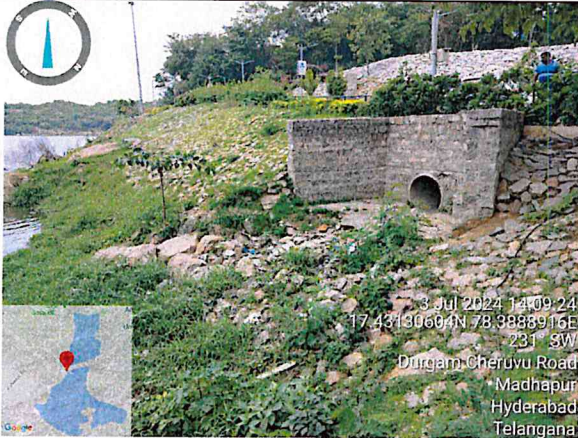
Durgam Cheruvu storm water drain inlets
