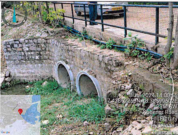
Durgam Cheruvu storm water drain inlets
